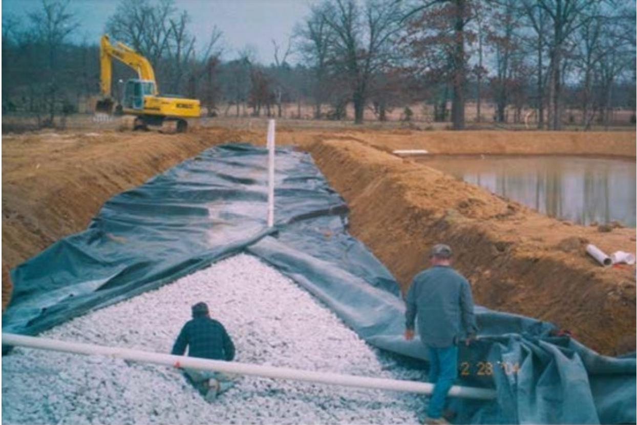
Figure 7: Long narrow ALD. Workers wrapping the limestone with synthetic liner before burial. Vertical pipes are used to measure head loss caused by the gradual accumulation of precipitate within the porosity of the limestone.
