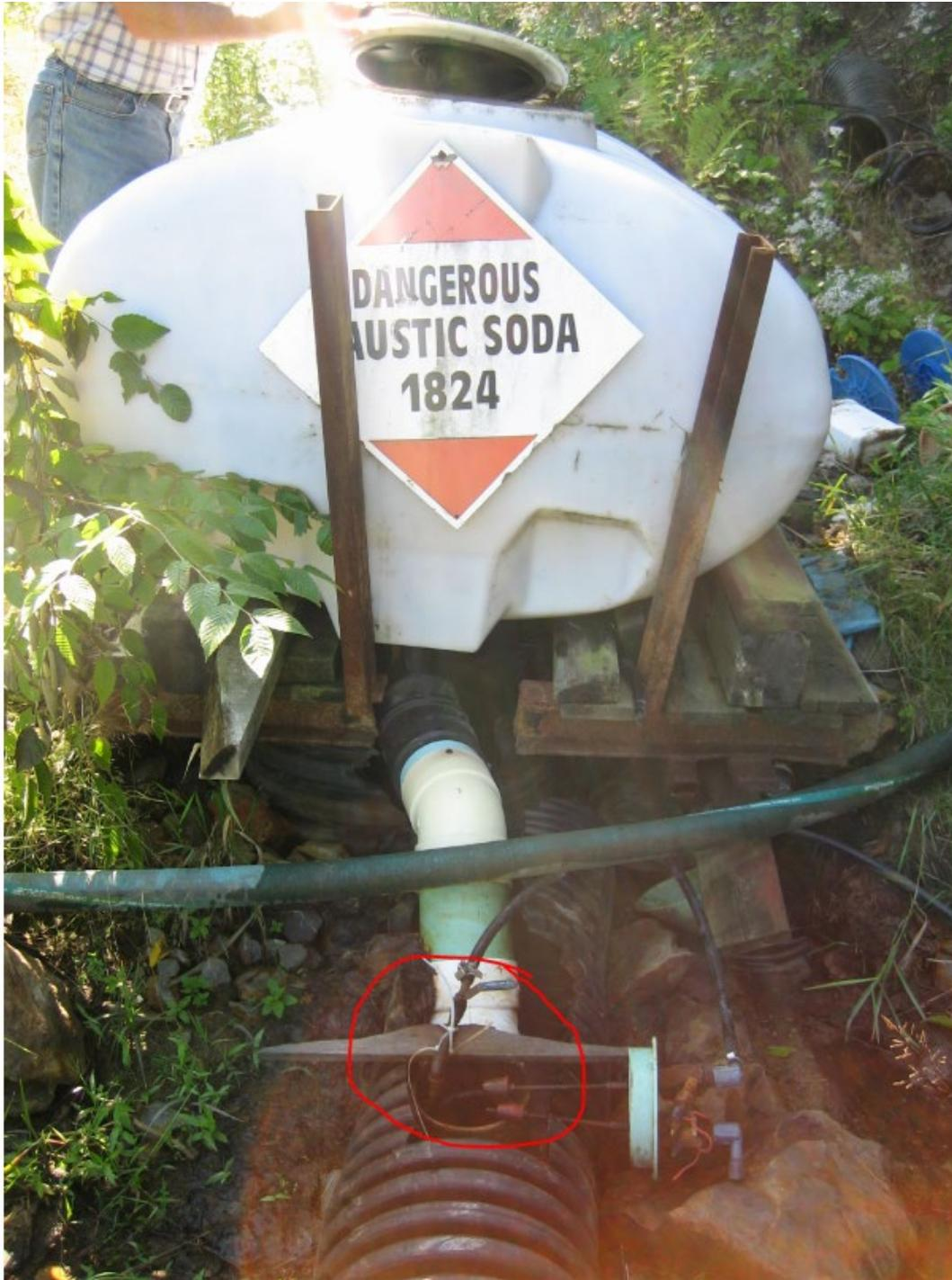
Figure 7: Photo of a 500-gallon poly tank. Mine drainage is in the black corrugated pipe and is dosed with Caustic Soda at the area circled in red.
