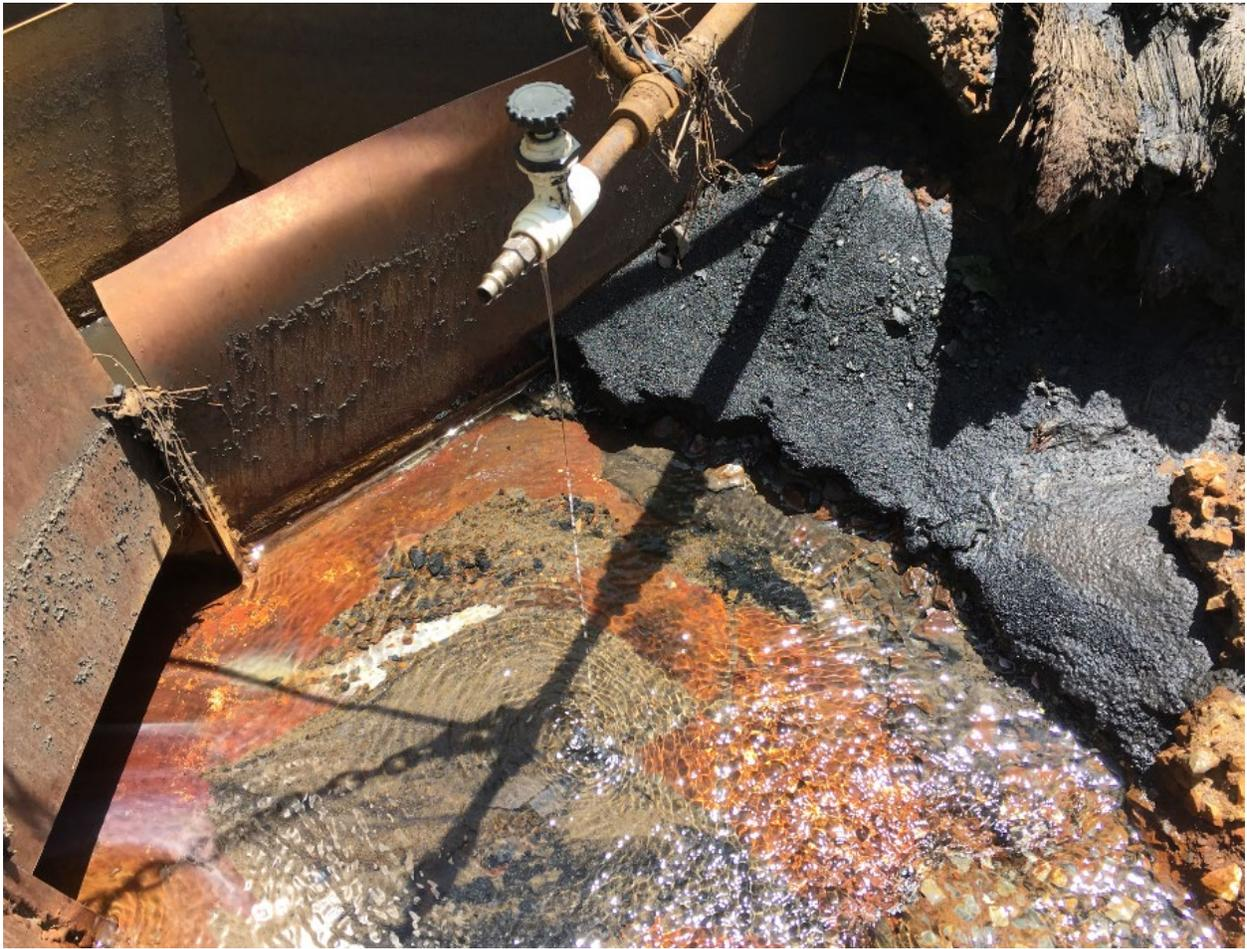
Figure 13: Another example of a needle valve being used for precise control of Caustic Soda dose.
