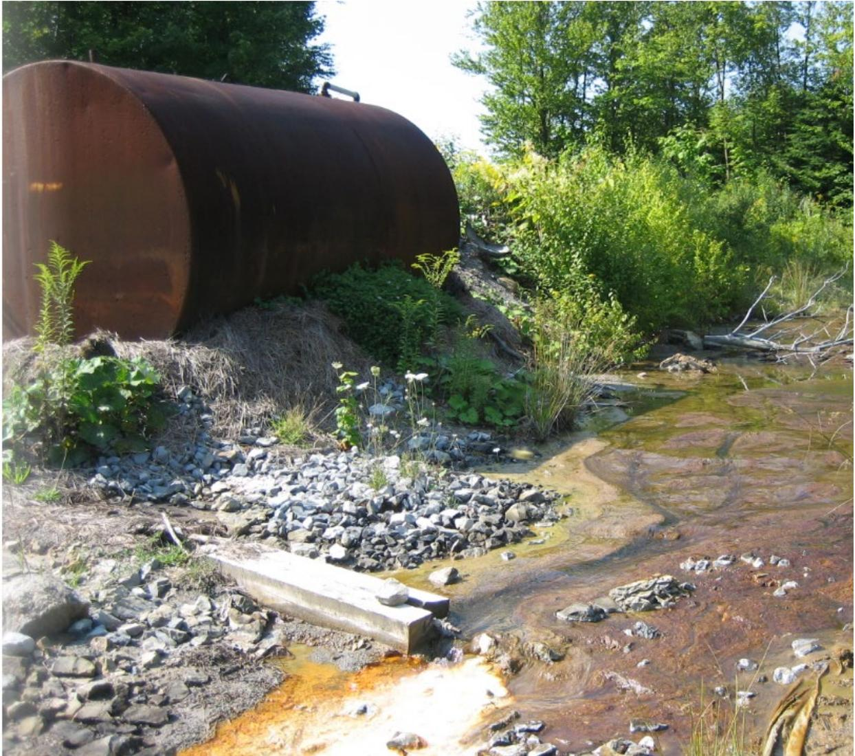
Figure 9: A steel tank capable of accepting bulk deliveries of Caustic Soda. A dosing line and valve are secured in place by a wooden trough. Note the whitish-colored aluminum hydroxide precipitate forming at the point of addition, which illustrates the quick precipitation reaction.
