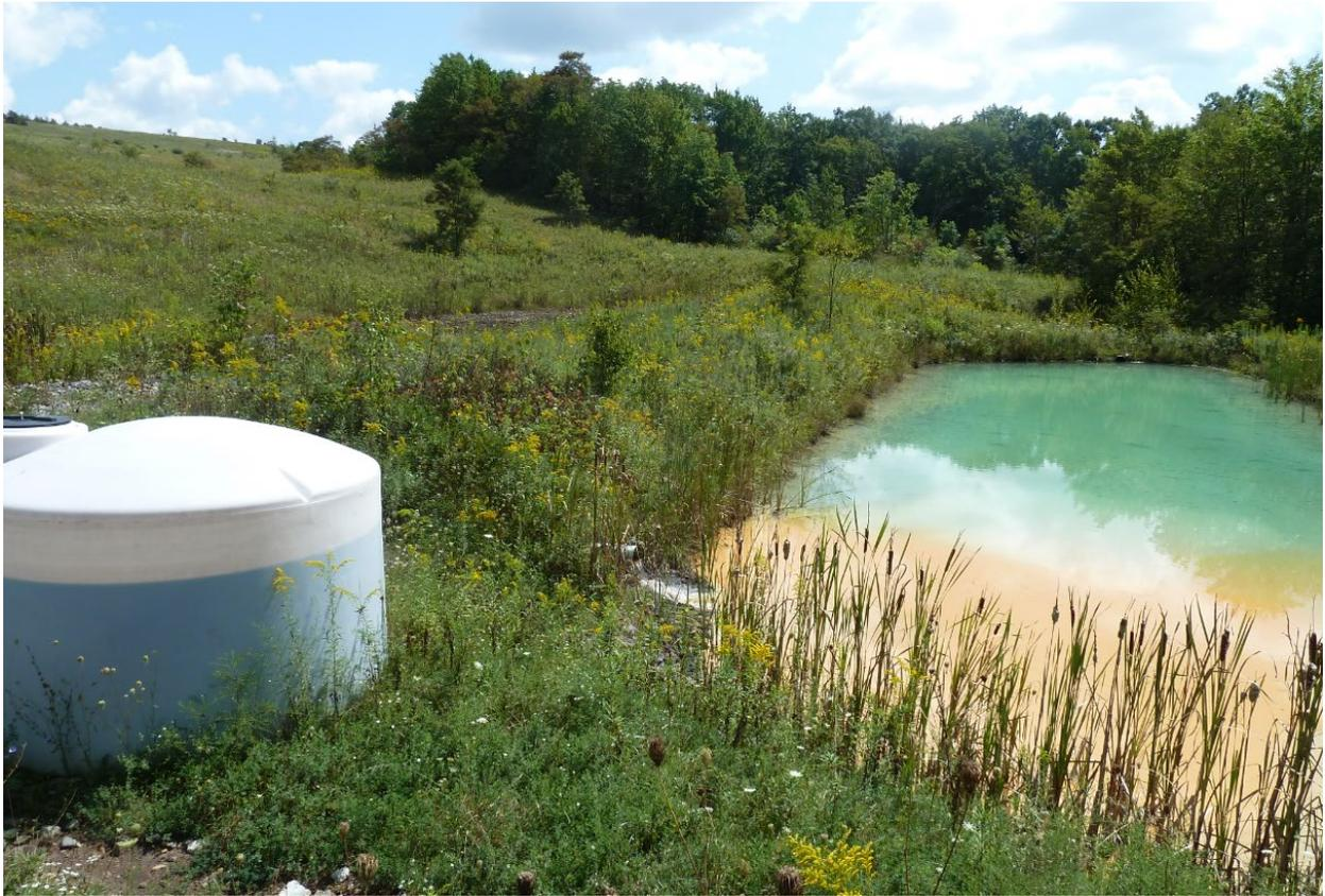
Figure 6: Photo of a 2,500-gallon poly tank filled with 20% NaOH. Note the fill level can easily be seen through the poly tank. The unit cost of Caustic Soda will be more since this is less than a bulk delivery. Having two sites that use 2,500-gallon tanks will allow for a split delivery to obtain optimal pricing.
