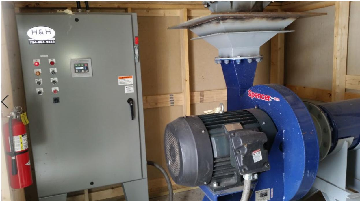
Figure 23: Spencer blower and electrical panel with variable frequency drive control panel inside of building shown in Figure 22.
