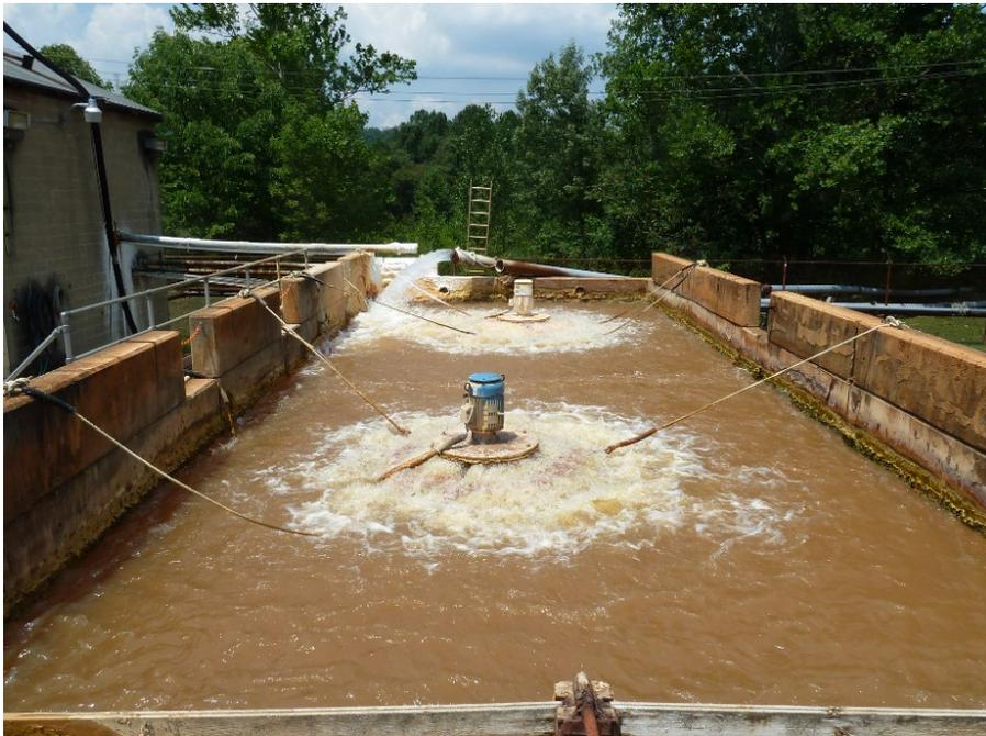
Figure 8: Two surface aerators in a plug flow reactor providing decarbonation.
