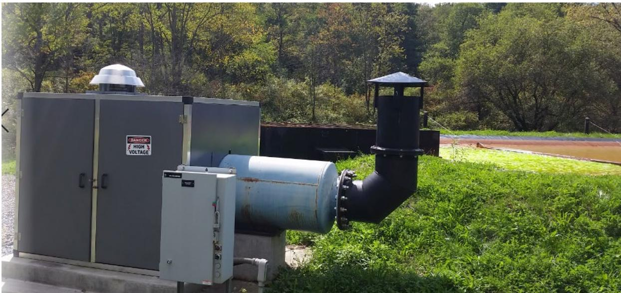
Figure 17: Compressed air blower housed in acoustic-silencing housing. Maelstrom is located in a residential area and noise was a concern. AMDTreat does not include the cost of acoustic housing.
