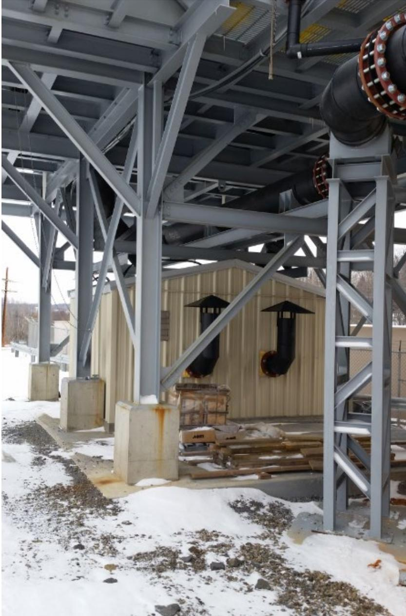
Figure 22: Sixty HP blowers enclosed in acoustic building to reduce noise. The Maelstrom Tanks sit above the building on top of the steel structure.
