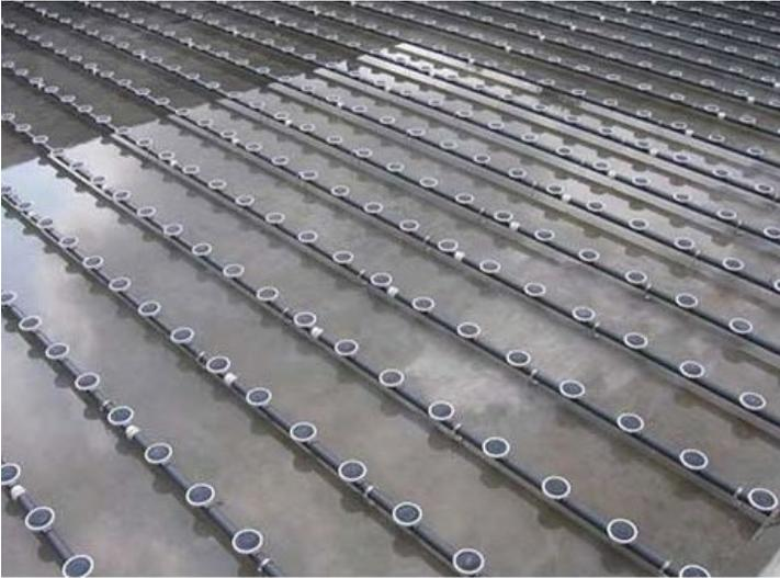
Figure 10: Fine diffuser aeration system with a piping grid at the bottom of a tank and disk diffusers.
