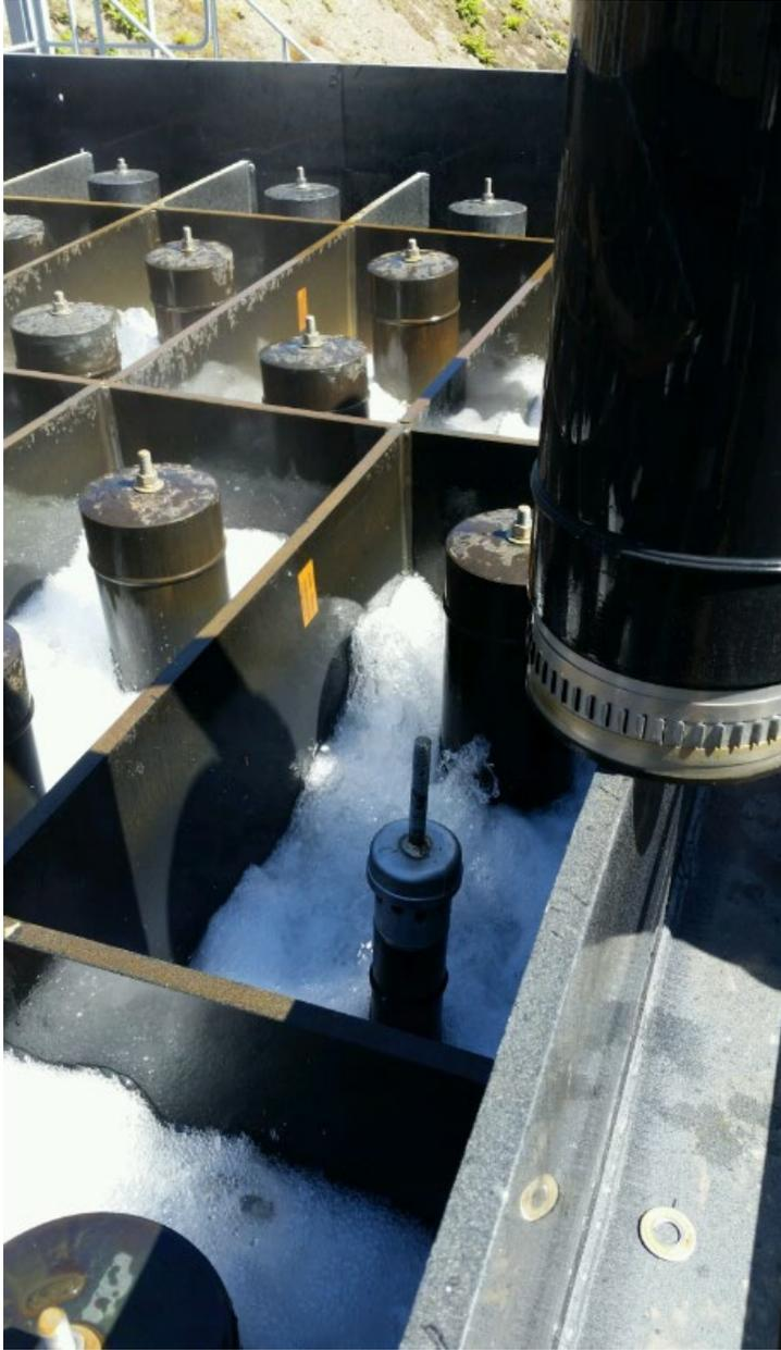
Figure 19: Photo showing the air tube (steel tube in tank) with air tube housing removed. Compressed air from the plenum flows to the top of the air tube and down in between air tube and housing before exiting through the stainless-steel air nozzle band.
