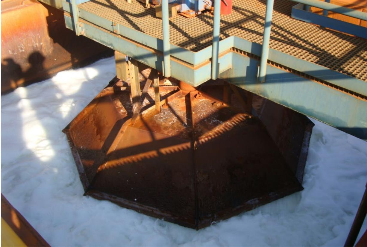
Figure 9: A surface aerator mounted in a continuous stirred reactor pulling water to the surface and creating droplets under the splash hood. Note the bubble froth promotes strong gas transfer, however, better results would be seen with froth in a plug flow reactor.
