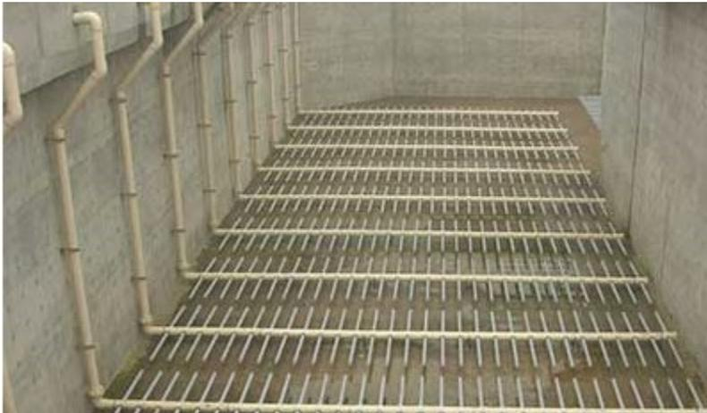
Figure 11: Fine diffuser aeration system with a piping grid at the bottom of a tank and tube diffusers.
