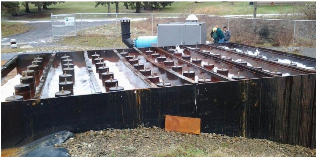
Figure 15: Maelstrom Oxidizer aerator unit. The blower enclosed in acoustic silencing housing is shown in the background and the aeration unit is shown in the foreground.
