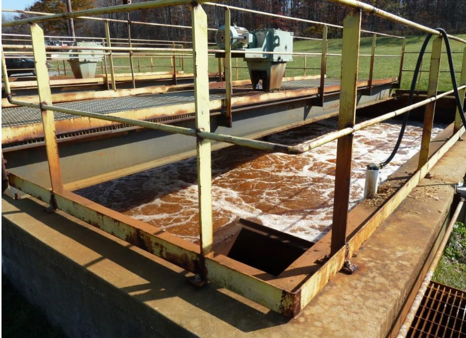
Figure 14: Fine bubble diffuser decarbonation system configured as a plug flow reactor.
