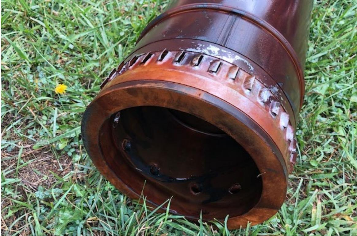
Figure 20: Air Tube removed for maintenance. The air orifices on the stainless-steel band at the bottom of air tube are pressure washed to remove scale and precipitate from clogging orifices. Note the orifices are directional and results in half of the air tube forcing air horizontally and countercurrent to the water flow. This causes strong mixing between water/air that is optimal for gas transfer.
