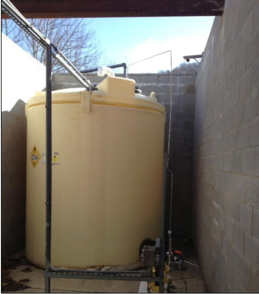
Figure 5. Photo of a HDPE Double-Walled dose tank.
