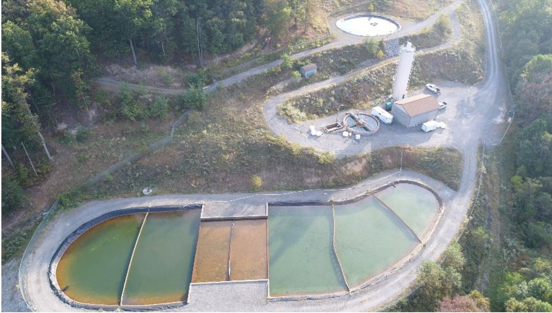
Figure 8: Floating baffles to promote settling of solids. The shallow narrow portion of the pond is to provide aeration and flow distribution as water flows through the pond.
