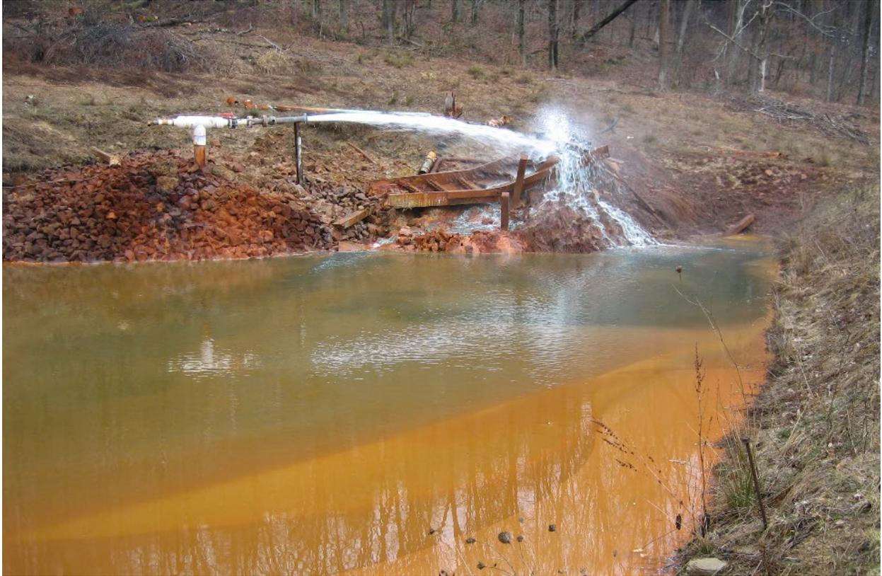
Figure 5: Pond with aeration (venturi) device at inlet of pond.
