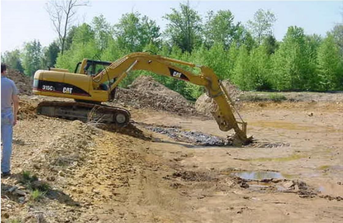
Figure 14: Photo illustrating the mechanical excavation of sludge from pond.
