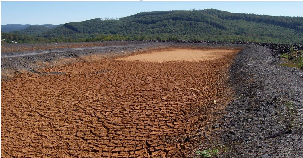
Figure 13: Drying bed being utilized to allow sludge to dewater and dry out.
