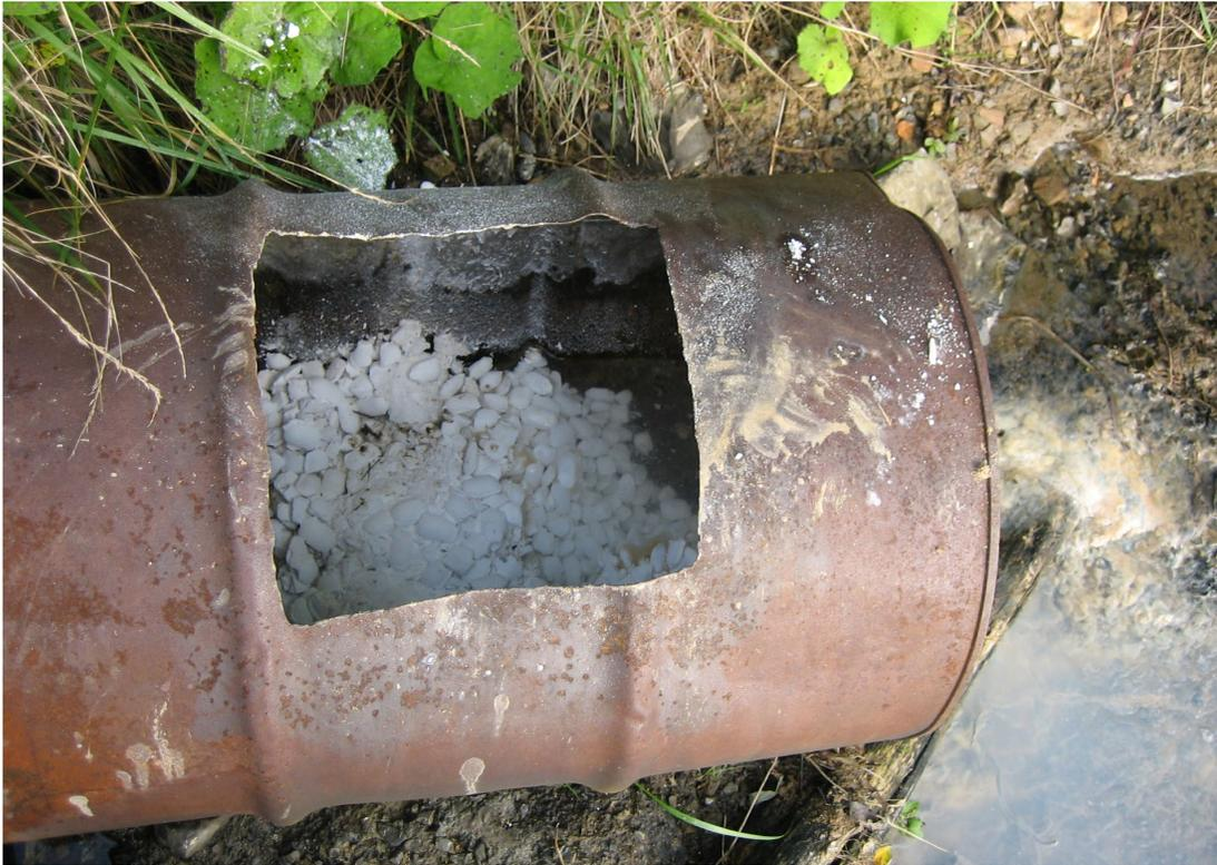
Figure 1: 55-gallon barrel with hole cut into it containing soda ash briquettes, with mine drainage flowing through each end of the barrel to allow dissolution of soda ash.
