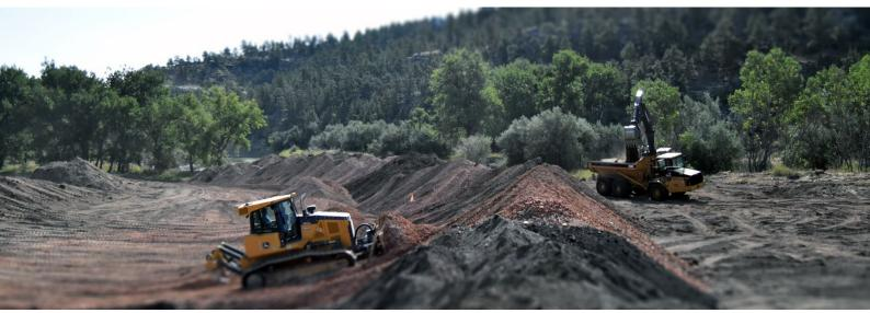
GPS-assisted equipment excavate approximately 47,500 cubic yards of material at the Bair-Collins Mine Reclamation and Floodplain Restoration Project in Roundup, Montana. Photo courtesy of Montana Department of Environmental Quality.
