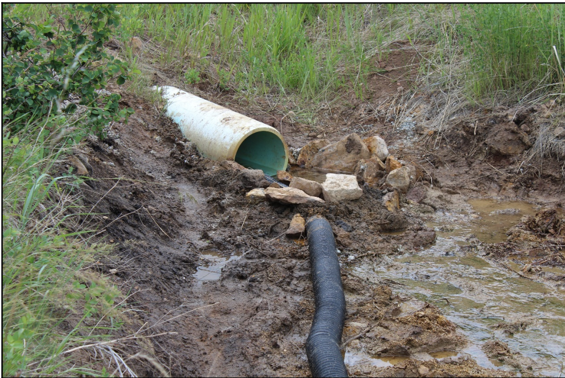
Figure 4.12: Dam constructed at ARD source to route ARD into gutter drain.
