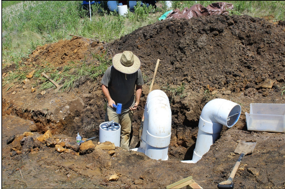
Figure 4.7: Fourth cartridge installation to the modular treatment system.
