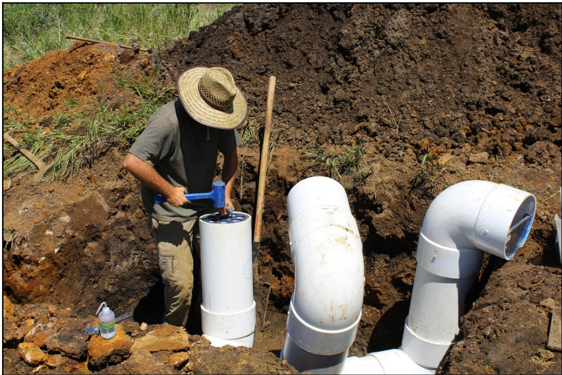
Figure 4.6: Third cartridge installation to the modular treatment system.
