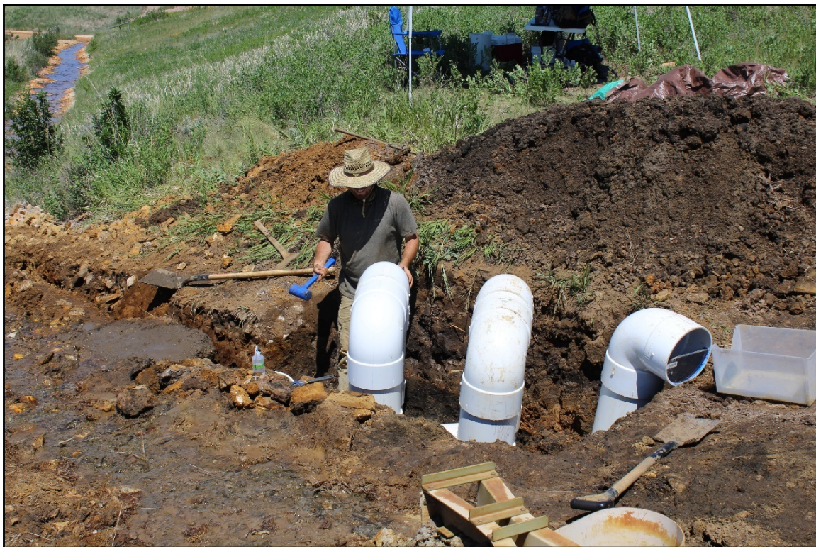
Figure 4.8: Fifth cartridge installation to the modular treatment system.
