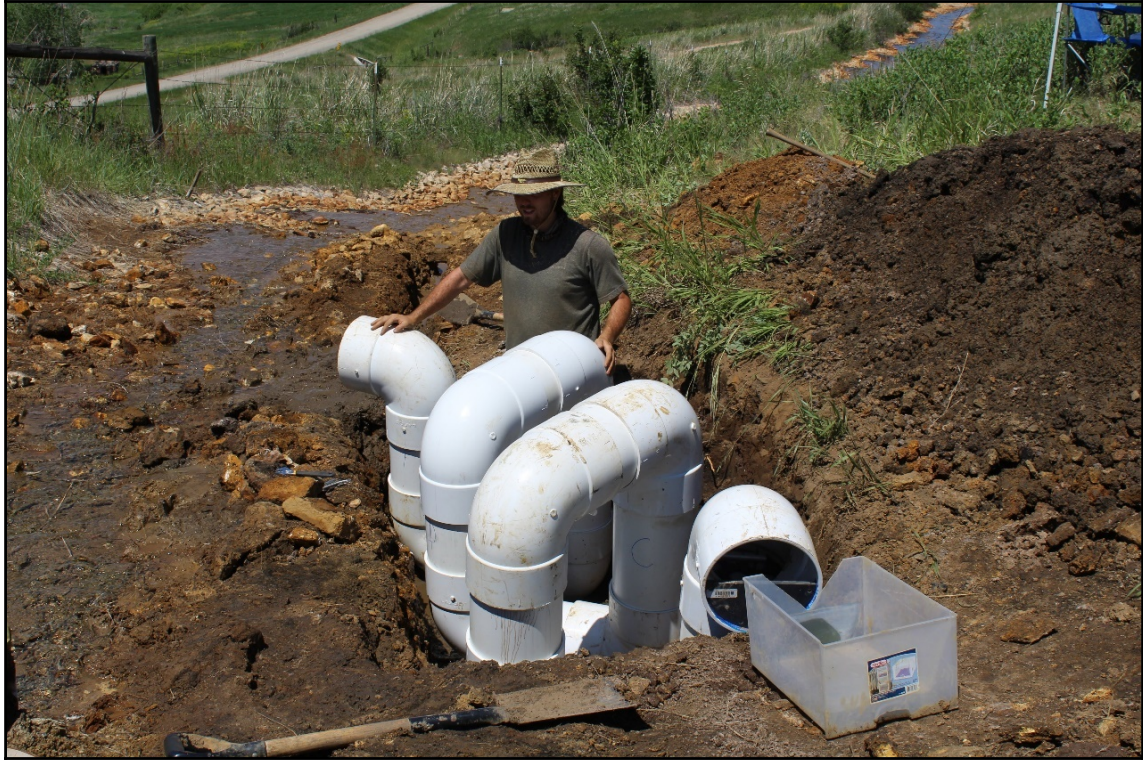
Figure 4.9: Sixth cartridge installation to the modular treatment system.
