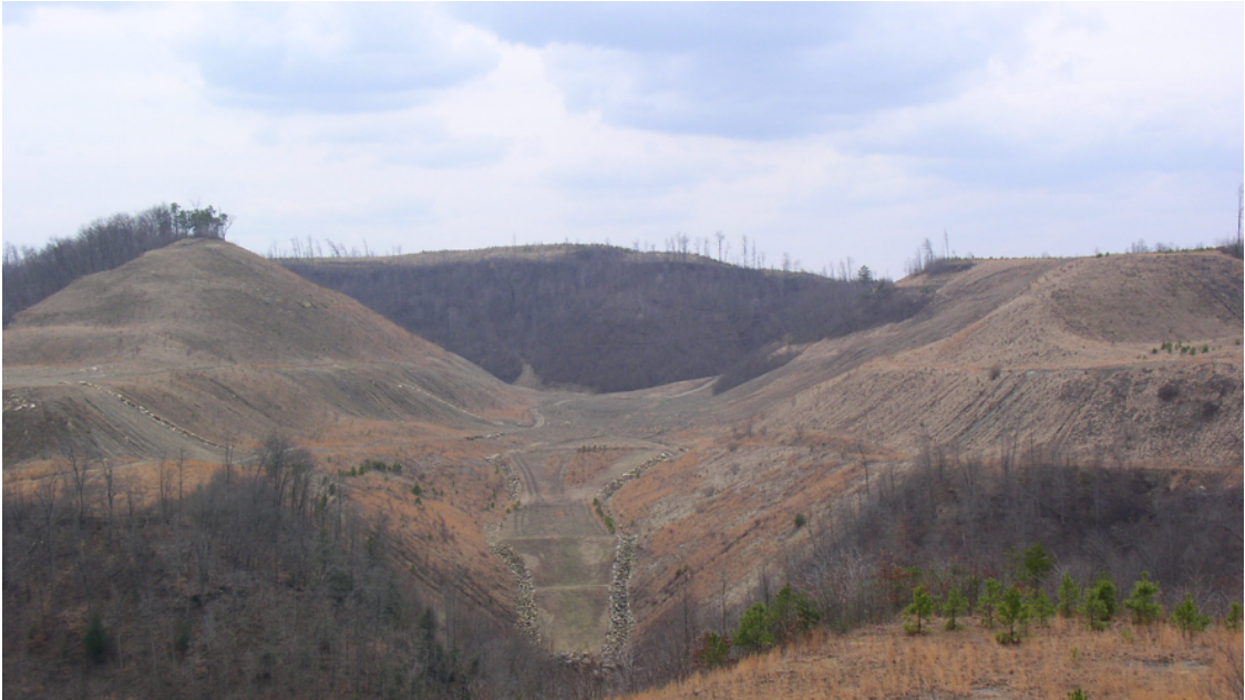
Figure 3.1. The Guy Cove valley fill in 2007, prior to creation of a headwater stream system. Note: forested section in the top center of the picture is an area that was not mined and where a small stream channel remained relatively intact.
