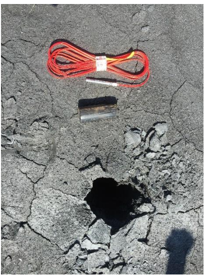
(a) A drilled hole and the explosives
