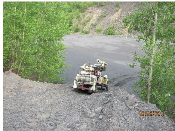
(b) The track rig was moving up a steep slope
