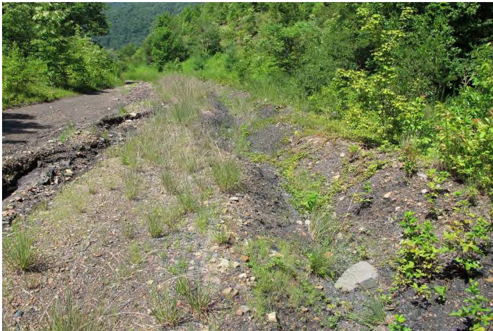
Figure 33. R070700 Access Road and vegetated contact ditch.
