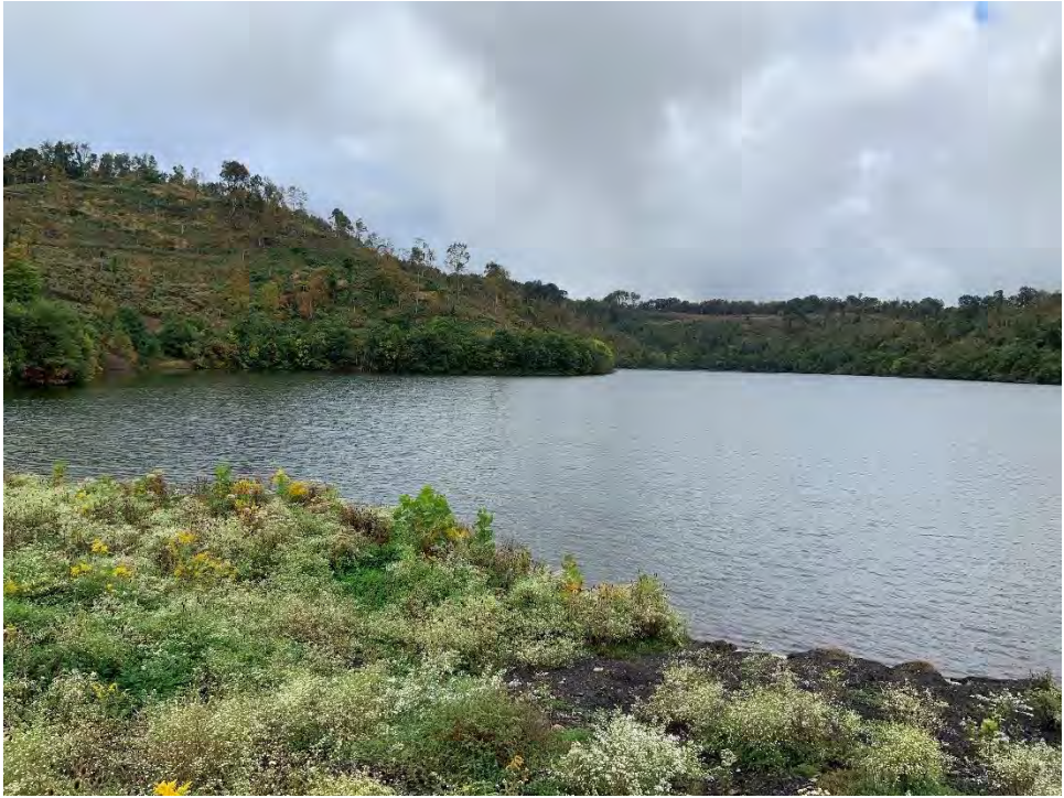
Figure 21. Slurry impoundment reservoir.
