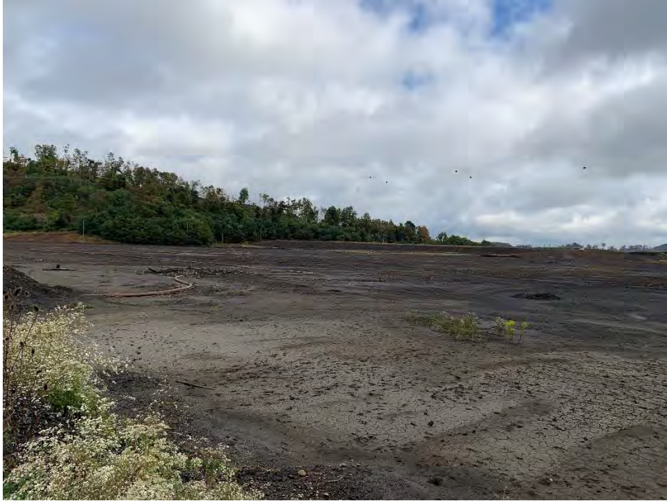
Figure 22. Beach of fine and course coal refuse pushout on upstream face.
