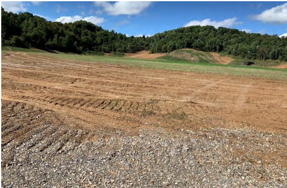
Figure 17. Filled-in slurry pool.
