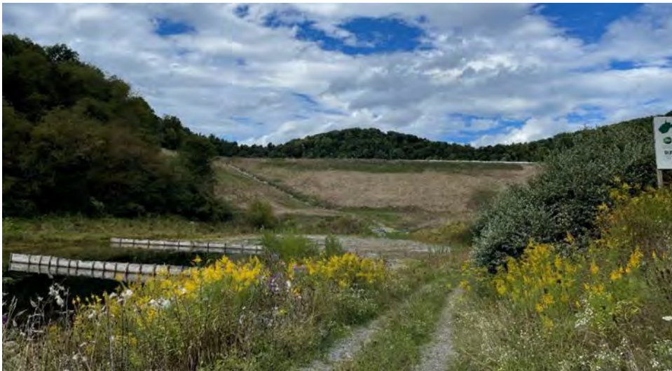
Figure 19. View of downstream embankment.
