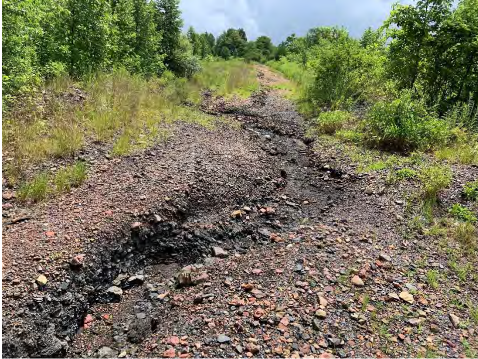
Figure 32. R070700 Access Road.
