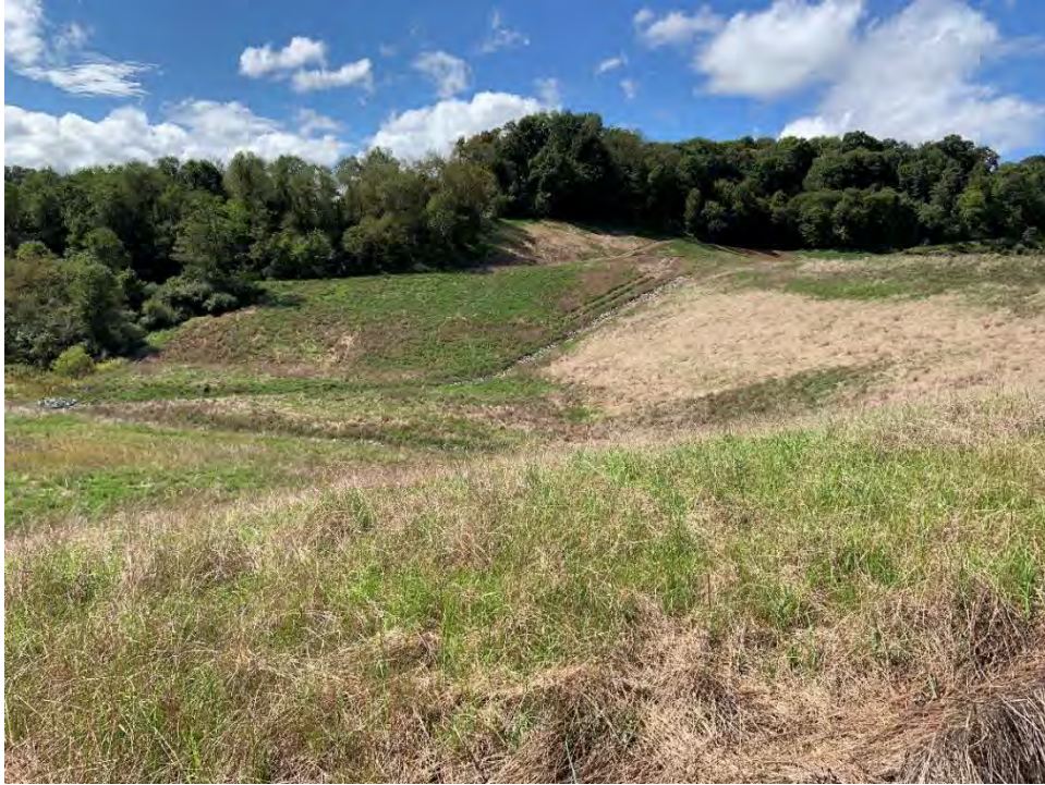
Figure 18. Reclaimed downstream embankment.
