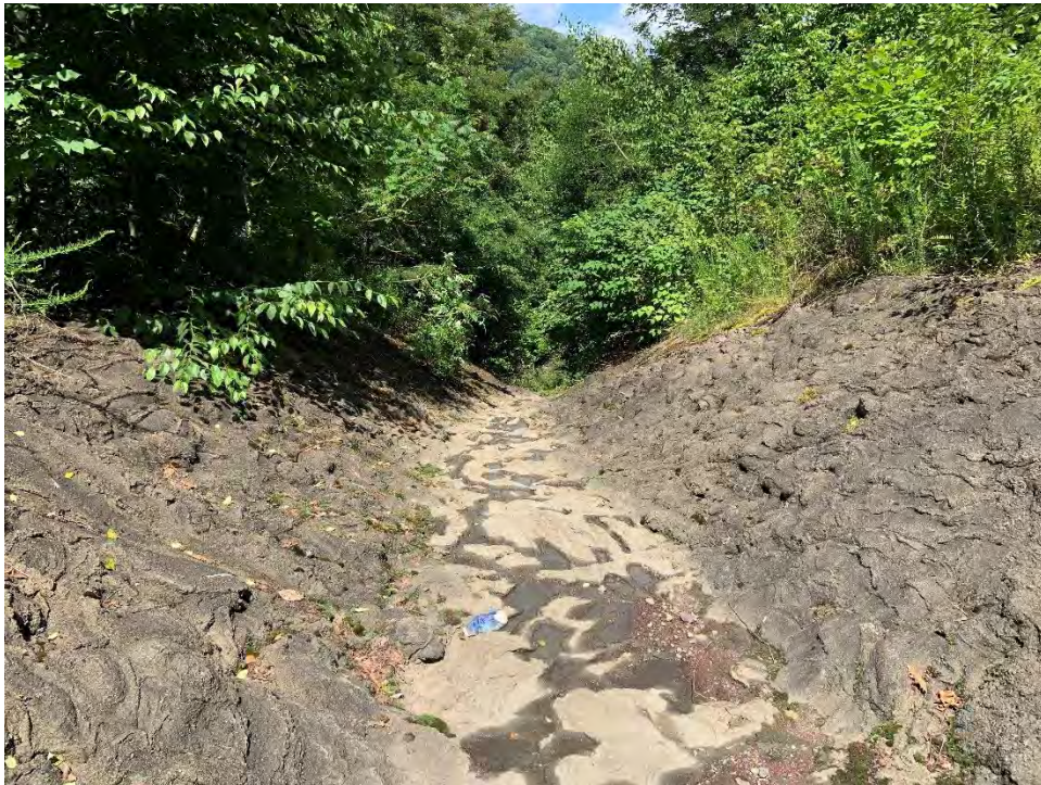
Figure 35. R070700 Grouted riprap.
