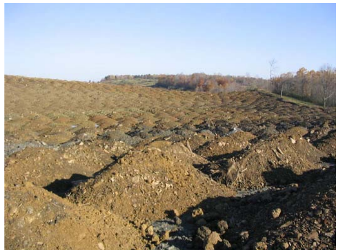
Photo 2. Loose-dumped soils on the surface at an Ohio mine site.
