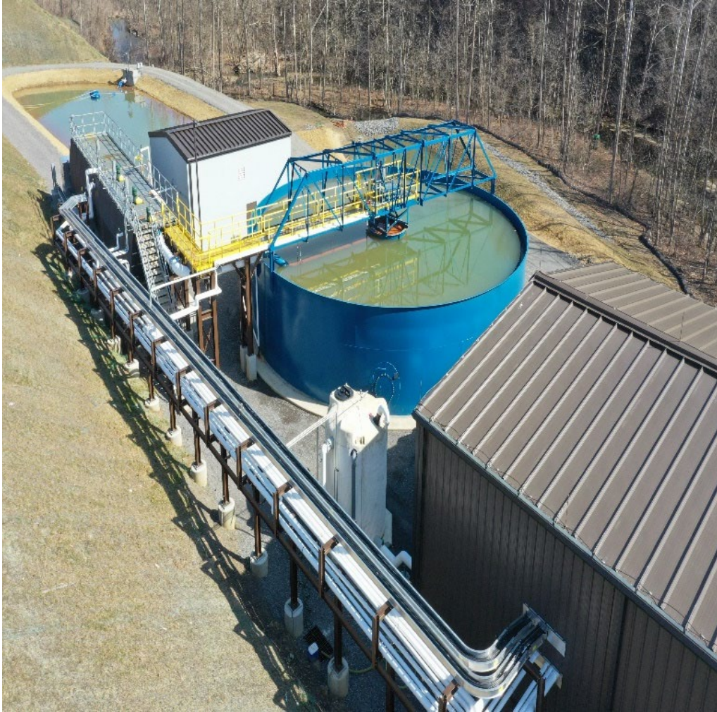
Gladden AMD Control Building, Clarifier and Polishing Pond Photo Credit: Pennsylvania Department of Environmental Protection
