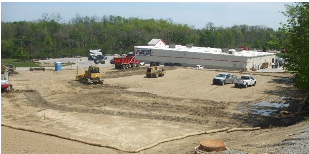
Final site grading after Cadiz CIC project site was compacted Photo Credit: Ohio Department of Natural Resources
