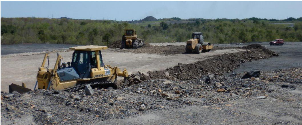
Reclaimed area being compacted at the Audenreid Coal to Solar Site Photo Credit: Pennsylvania Department of Environmental Protection
