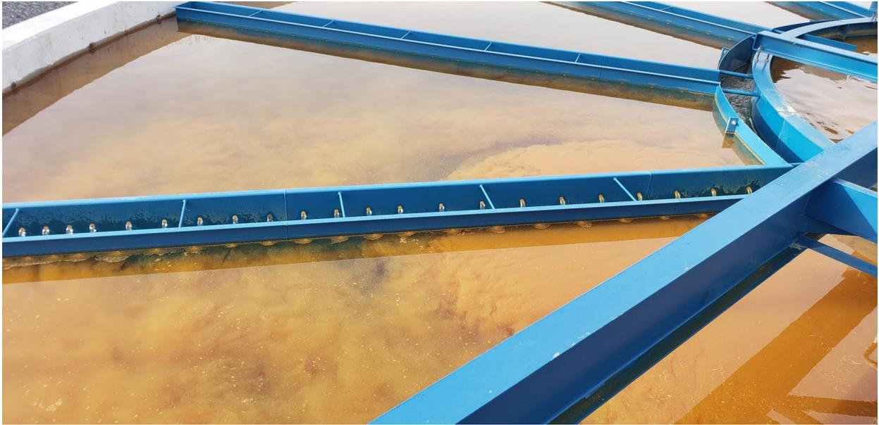
Figure 13: Photo of a disrupted clarifier discharging the sludge blanket due to an incorrect solids inventory handling plan. A change to both the elevation to maintain the sludge blanket and the sludge pumping schedule fixed the issue.
