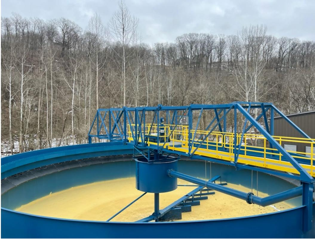
Figure 31: A newly constructed welded steel conventional clarifier with a concrete floor. Note the greyish density curtain baffle extending the perimeter of the inside wall under the laundering weir.
