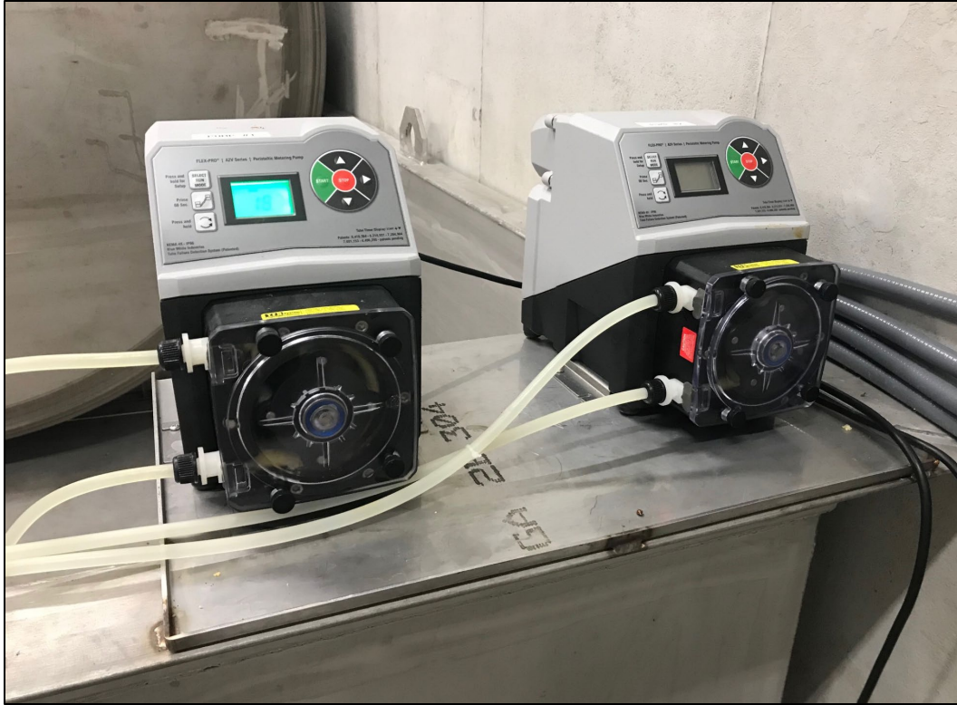
Figure 10. Photo of a two-pump hydrogen peroxide dosing skid and associated polyethylene tubing. Note these peristaltic pumps have automated leak detection systems that will stop the pump in the event of a tubing failure.
