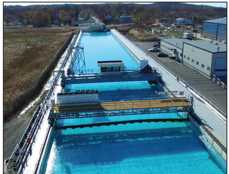
During the 25 years of BSEE oversight, the Ohmsett facility has been a test bed for innovative technologies for oil spill response.
