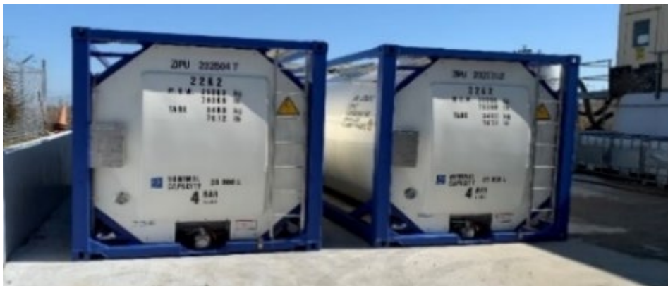
The MC20 oil is now stored in two ISO tank containers that are in the secondary containment adjacent to the Ohmsett tank.
